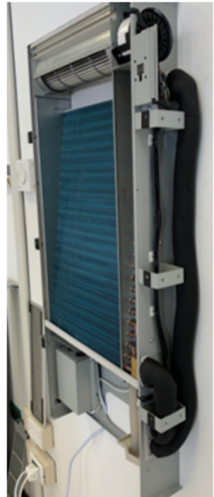
PUT INSULATION IN ALL THE EXTERNAL PIPE
