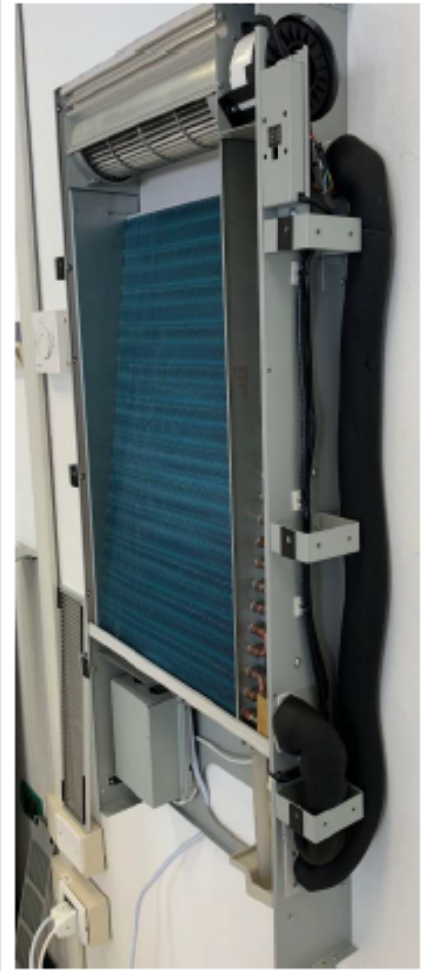
PUT INSULATION IN ALL THE EXTERNAL PIPE
