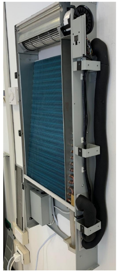
PUT INSULATION IN ALL THE EXTERNAL PIPE
